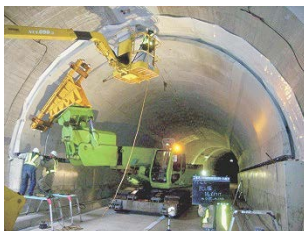
写真-4 PCL版設置
