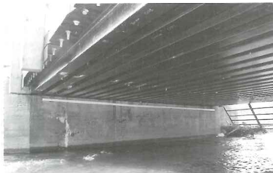
写真-1 Tom's Creek Bridge
